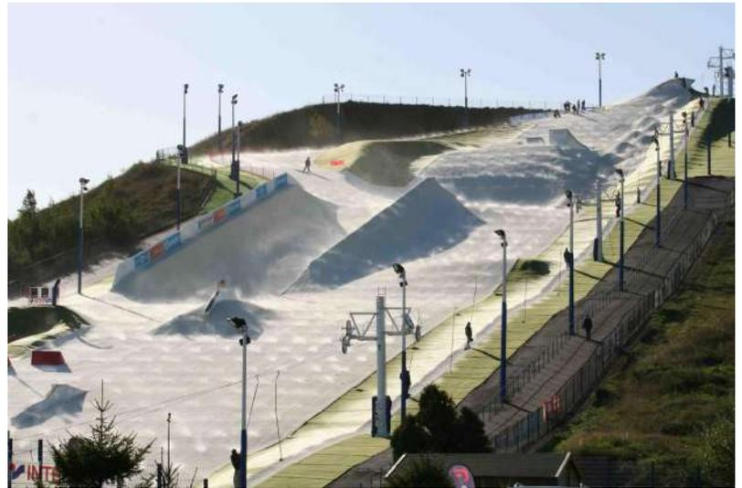
Again, please note how Briton Engineering designs Snowflex hills. From top to bottom, there is one main carpeted area of Snowflex material. In the second photo, you can clearly see the misters dotting the white astroturfing. This is how Snowflex works. It consumes a lot of water to
